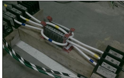
Figure 18 Common mode choke wound per manufacturer's instructions
